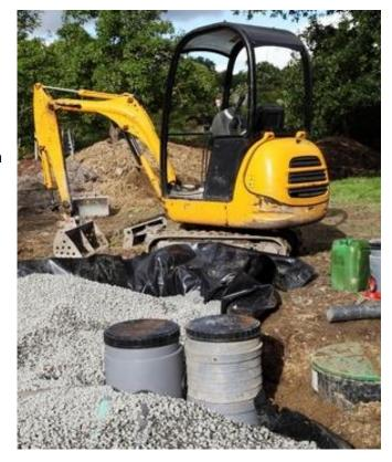
the ground, drainage capability of the soil as well as the types of load which may occur (if installed underneath a drive way or regularly driven area) must be checked prior to installation.
