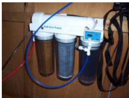
Figure 33 RO filter
