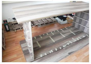
From underneath it, mark the places for the screws on the upper board and the second board:
