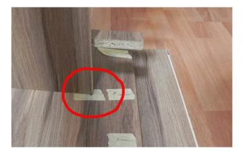
Use a cutter to cut the excess tape if it does not come off easily. Also, it is very important to remember not to place the brackets very close to the edge because they might get in the way of your cans:
