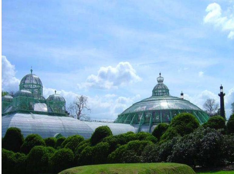
The Royal Greenhouses of Laeken in Brussels, Belgium.
